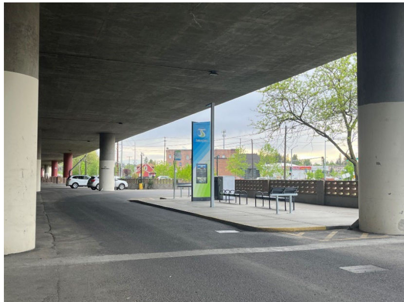
(Jefferson Street/I-90 Park and Ride HPT Stop Improvements)
