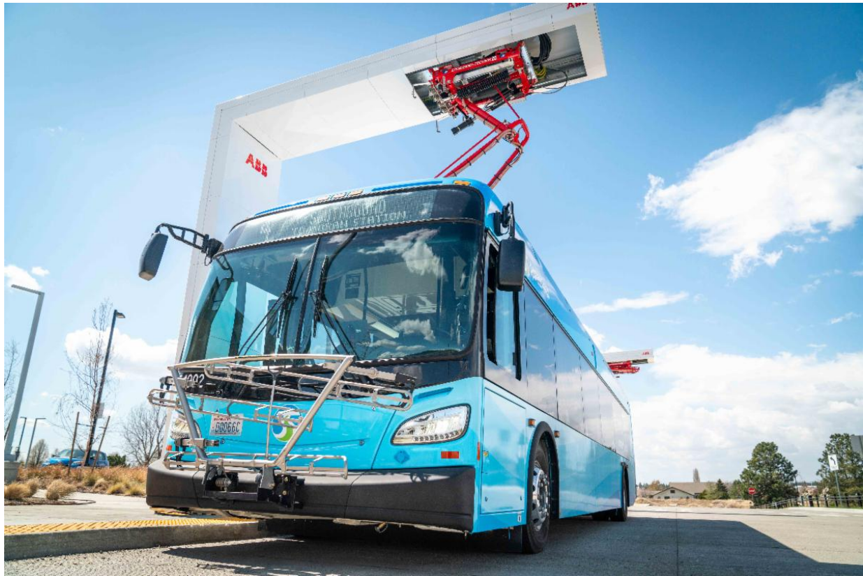
Above: STA's battery-electric bus being charged at Moran Station Park & Ride
