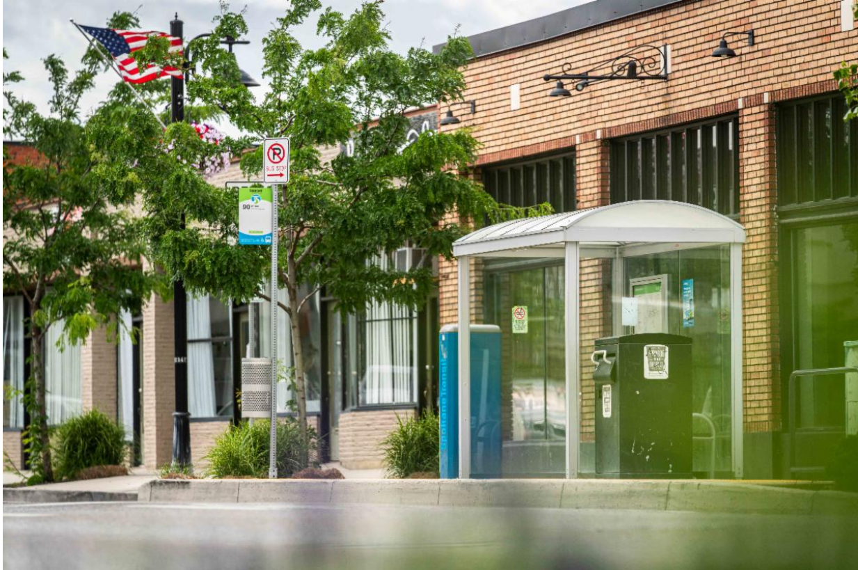
Above: An upgraded bus stop along Route 90 Sprague
