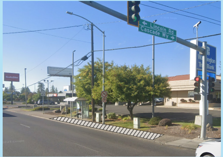
Street view of the station location (Google Street View)
